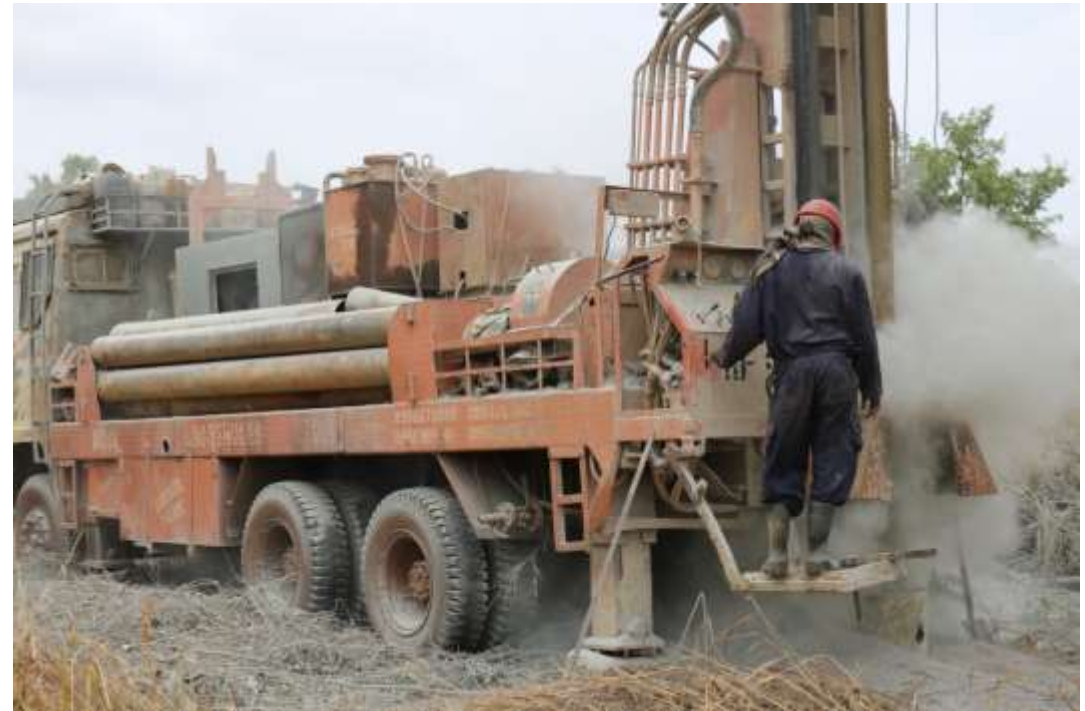
Digging for another well
